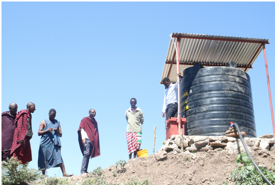
Figure 6: Water Filtration [completed Feb 2023]
