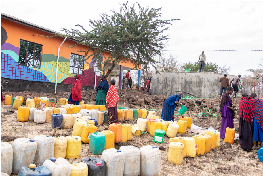
Figure 1: 100k Liter Water Harvesting Unit [Completed June 2022]
